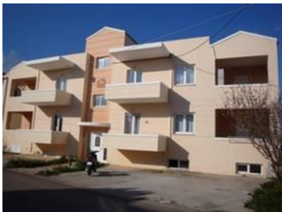
View of the apartments
